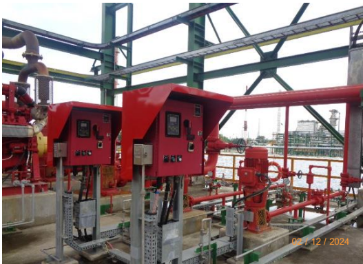
Electric Motor Driven Jockey Pumps
