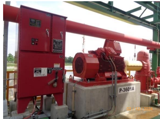
Electrical Driven Fire Water Pump
